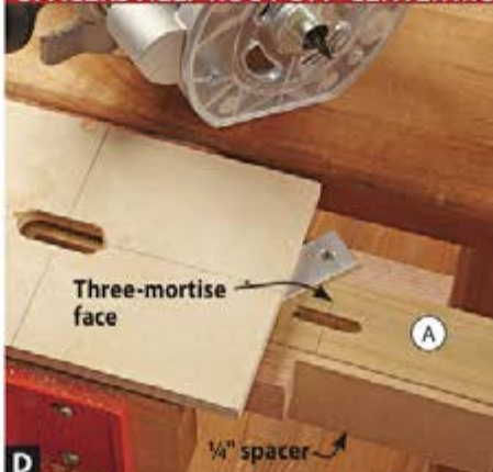
D To offset from center the mortises on the three-mortise face of each leg, position a \frac{1}{4} " spacer against the tapered face of the leg.
